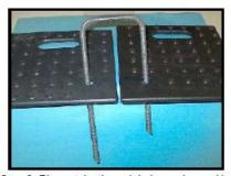
Step 3: Place stake through holes and pound into soil using Sledge Hammer.
