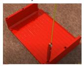
1) Always install/remove the system from a position of safety. Place a Manholebox panel on its back and carefully lower the assembled strut into the strut pockets using a suitably rated shackle.
