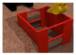
7) Using the excavator bucket, dig and gently push down each corner of the Manholebox about 300mm increments. Take care to avoid damage to the panels.
