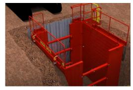
15) To close off the open edge of the Manhole walls, Trench sheet or edgesafe panels can be used. Using the excavator quick hitch, gently push on the Manhole sheet until it has reach the required depth.
