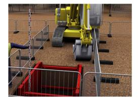
9) Operative to check the correct dig depth. Approximately 200mm upstand of the box is recommended before a top box is installed.
