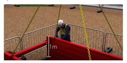
4) Operatives on even ground to remove chains only if the box upstand is 1m above ground level
