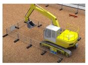
1) Mark out the digging area. Place pedestrian barrier around the excavation area. Start with 1m depth
