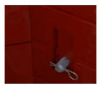
11) Operatives behind the pedestrian barriers to attach the top to the base using pins from outside and r-clips from inside of the Manhole box. Always ensure a safe and secure means of access prior to entry
