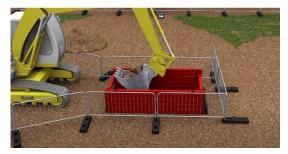
5) These barriers are temporary control measure to highlight the open excavation hazard
