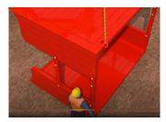
4) Using an excavator gently lower the second Manhole box panel over the struts and secure using pin and r-clips
