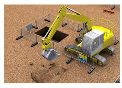
2) While digging, the spoil must be located away from the excavation and its zone of influence.
