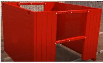
5) With the box laying on timber skids on stable ground, attach a two-leg chain to the handling point of the upper panel and using an excavator orientate the Manhole box into vertical position
