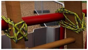
16) If a ladders safe platform is required, lower the platform over the Manholebox panel and secure with pin and r-clips.
