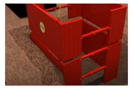
10) Using an excavator, lower the top onto the base using connection points. Marwoods do not recommend that more than 2 Top units be used with any one Base unit.
