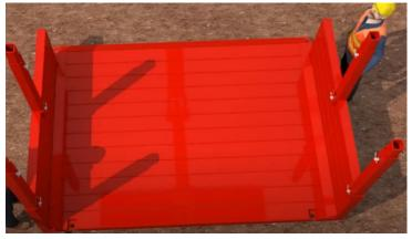
3) Attach the remaining struts into the three remaining pockets on the Manhole box panels
