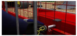
14) Behind pedestrian barriers, two operatives attach edgesafe and secure with clips and r-clips
