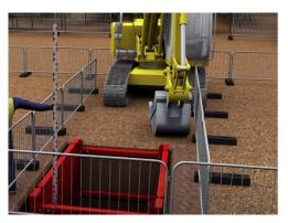
9) Operative to check the correct dig depth. Approximately 200mm upstand of the box is recommended before a top box is installed.
