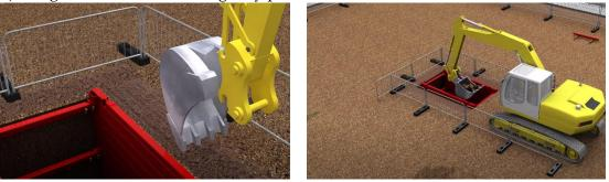
8) Level off ground prior to movement of pedestrian barriers.
