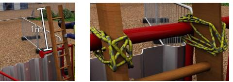
18) The ladder must be 1m beyond the ladder pole. Secure the ladder with a minimum 3m of rope
