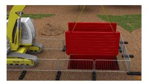
10) Using an excavator, lower the Trenchbox top onto the Trench box base. Marwoods do not recommend that more than 2 Top units to be used with any one Base unit.
