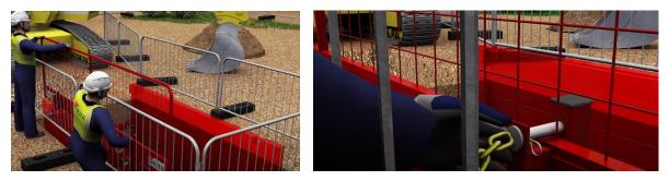
14) Behind pedestrian barriers, two operatives attach edgesafe and secure with clips and r-clips
