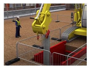
15) To close off the open edge of the trench walls, trench sheet or edgesafe panels can be used. Using the excavator quick hitch, gently push on the trench sheet until it has reach the required depth.
