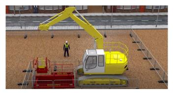
17) If a ladder safe platform is required, lower the platform over the Trenchbox panel and secure with pin and r-clips.
