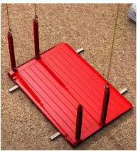
3) Attach the remaining struts into the three remaining pockets on the Trench box Panels.
