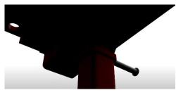
4) Using an excavator gently lower the second Trench box panel over the struts and secure using pin and r-clips.
