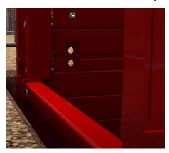
11) Operatives behind the pedestrian barriers to attach the top to the base using pins and rclips, either side of the Trenchbox.
