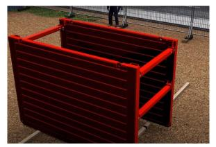
5) With the box laying on timber skids on stable ground, attach a two-leg chain to the handling point of the upper panel and using an excavator orientate the Trench box into vertical position as shown above.
