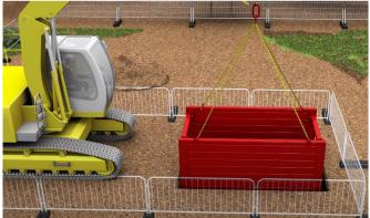
3) Lower the assembled Trenchbox into the excavation.
